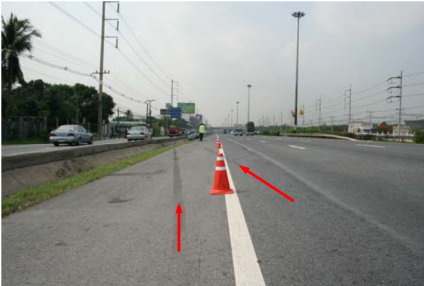
Figure 2: Crash Scene showing the Tire Marks of Running-off Road
